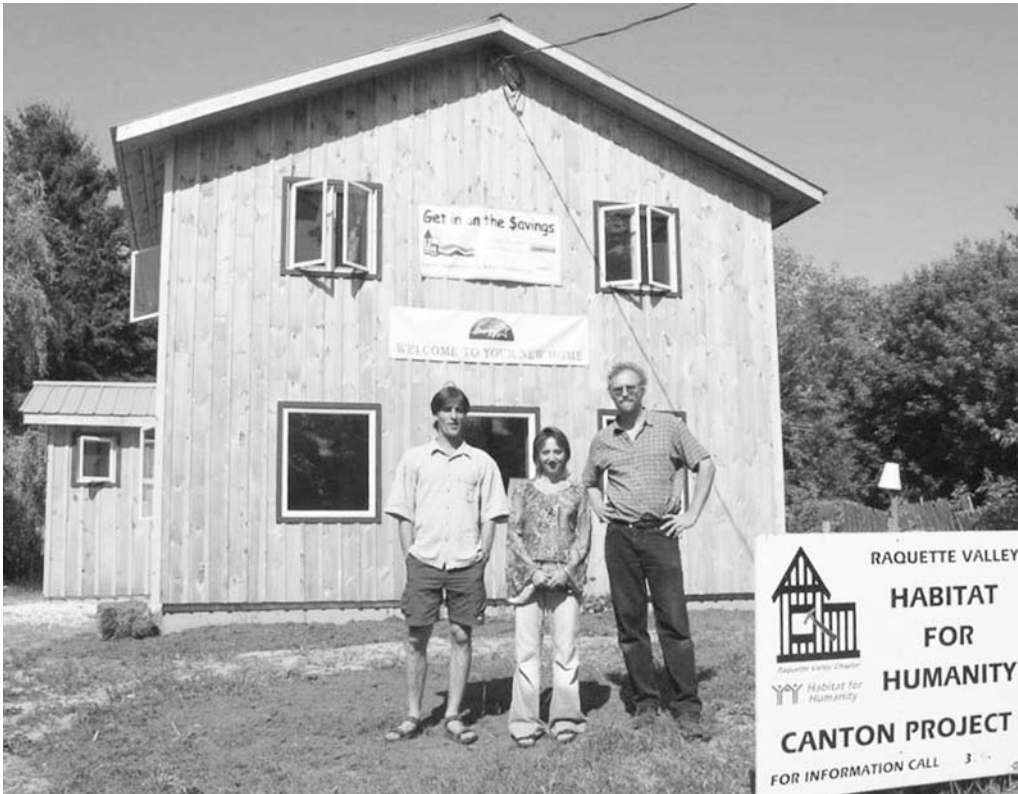
Standing in front of the completed home are builder Eric Schulze (left), owner Jennifer, and Scott Shipley. The final HERS rating score for the affordable and energy-efficient home was a gratifying 92.
