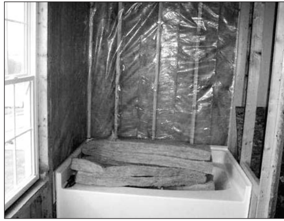
(left) A dropped soffit in a kitchen can funnel huge volumes of air if left unsealed from the wall and ceiling framing. (right) Here, the builder has provided a continuous air barrier on the outside walls before installing the tub.
