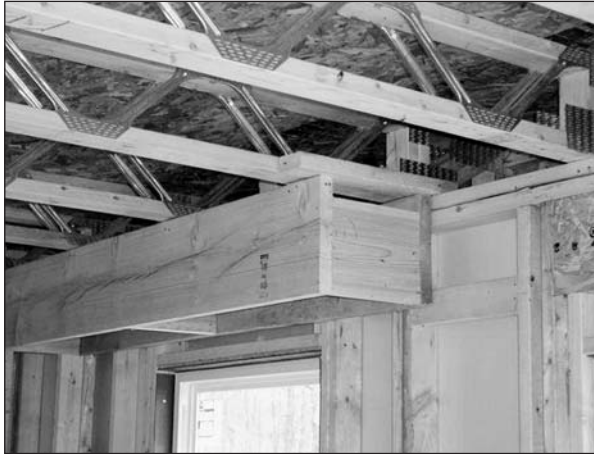
(left) A dropped soffit in a kitchen can funnel huge volumes of air if left unsealed from the wall and ceiling framing. (right) Here, the builder has provided a continuous air barrier on the outside walls before installing the tub.
