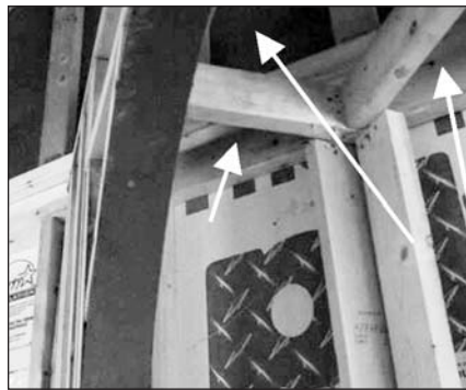
Note the opportunities for massive amounts of air leakage to the attic from within the fireplace framework.
