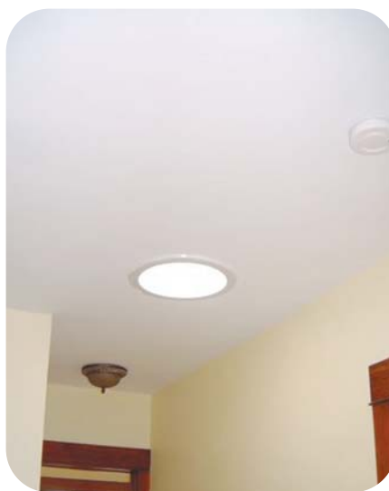
Tubular skylights have made it easier and less costly to bring natural light into a building.
