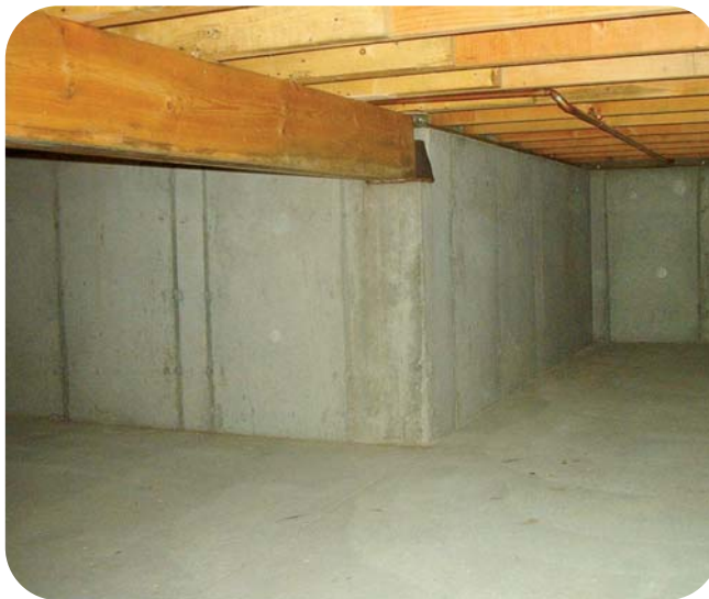
A sealed and insulated crawlspace with a vapor barrier on the floor has many advantages over the traditional vented crawlspace; it’s dry, and energy losses are minimal.
