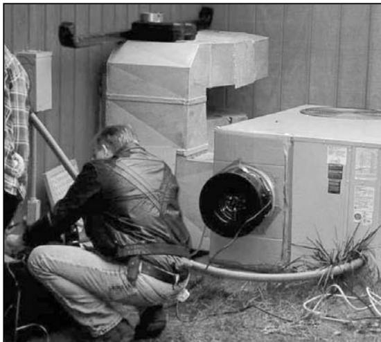
You never know what you may find in a client's home—even commercial package units such as this one can turn up in residential buildings.
