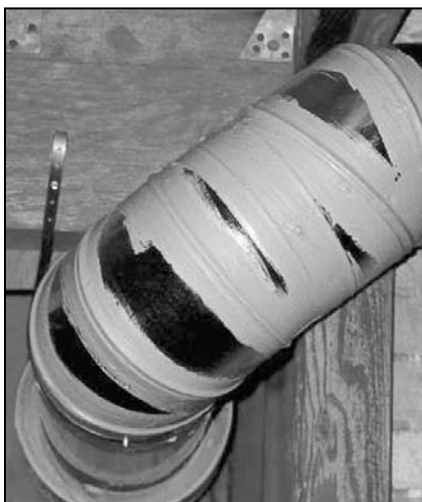
This is one well-sealed elbow.
