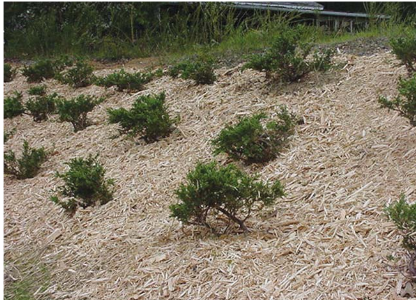
If you can grind your wood waste into 2 1/2-inch “minus” (meaning less than or equal to) wood chips, it makes a great soil erosion control mat.
